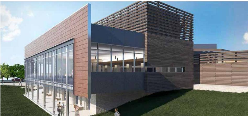
The University of North Dakota’s Wilkerson Commons, set to reopen this year, incorporates a terra cotta rain screen system integrated with a Hunter Xci Polyiso-based continuous insulation solution. Rendering courtesy of SCB.
