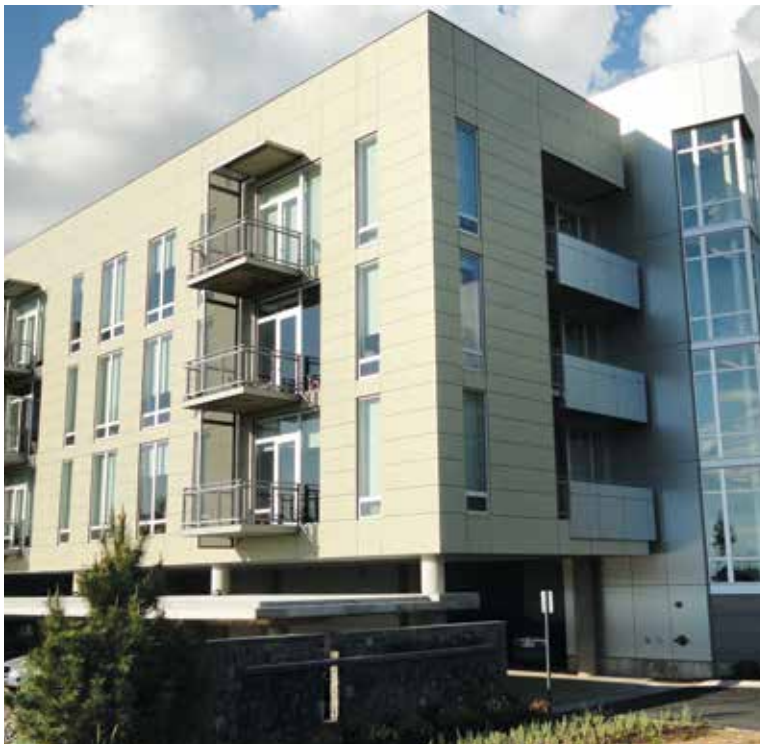
HHMI Research Campus - Ashburn, VA / WDG Architects
